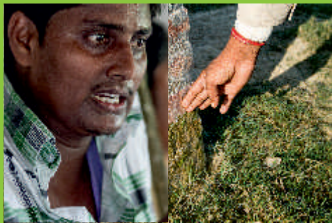
Kamal Kamat, showing where the plinth of their school would have been if the SDMC / VDMC had not intervened.
